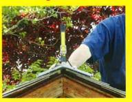
With the center bar pointing up, lower both wings to touch the roof on each side of the ridge. Read the pitch on the center bar.
