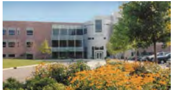
Parker Hannifin Corporation Headquarters Cleveland, Ohio
