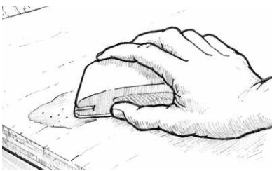
Figure 23 Sand cured fairing compound to desired contour.
