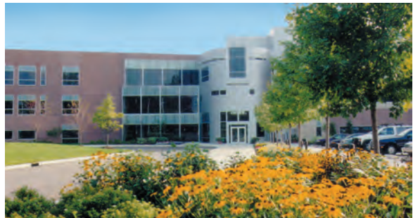
Parker Hannifin Corporation Headquarters Cleveland, Ohio
